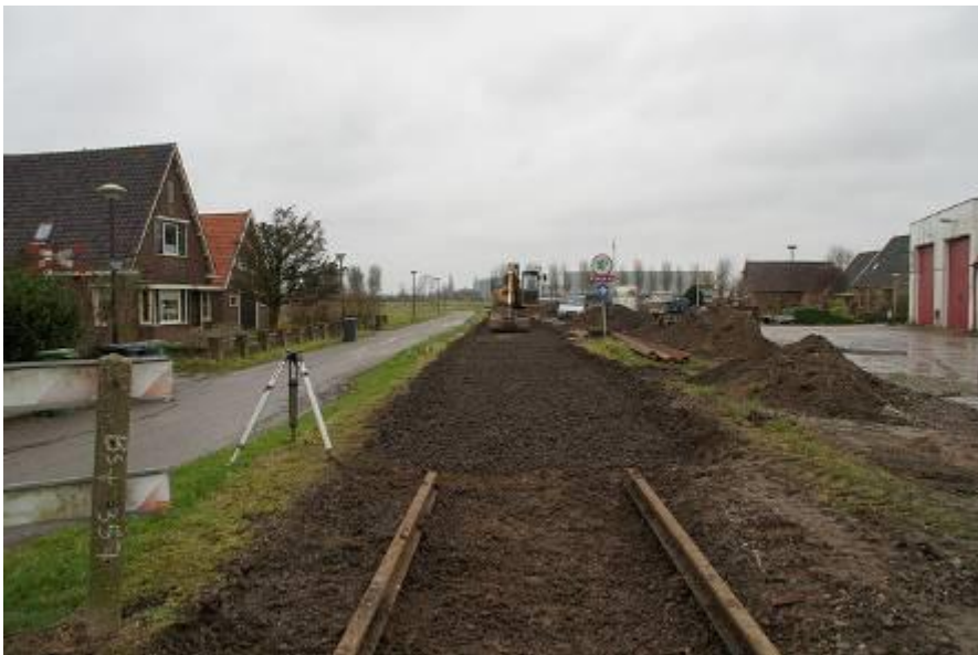
23 december 2011: spoorvernieuwing nabij Opperdoes.
