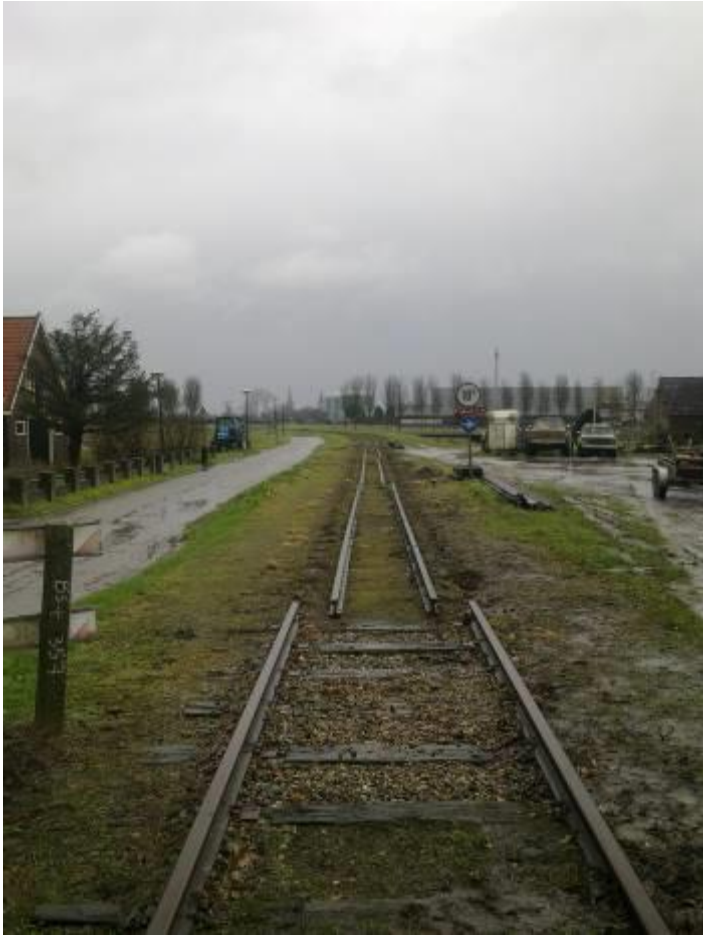
15 december 2011: spoorvernieuwing nabij Opperdoes.
